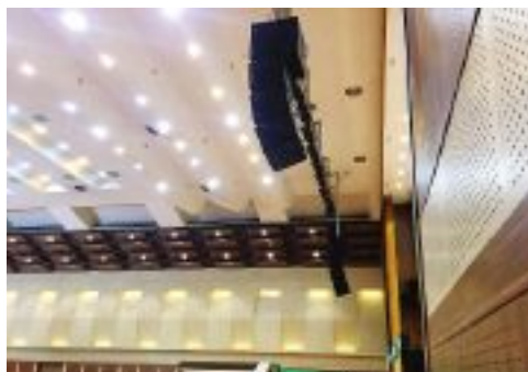
L-R hangs of Audac FX3015 tops and FX1.18 subs in the concert hall
