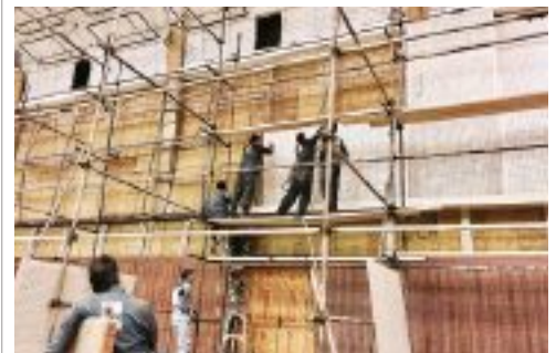
The team installed acoustic panelling in the concert hall
